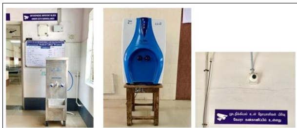
Fig 12: 24 hours RO water system, Hot water facility and CCTV facilities at wards.
